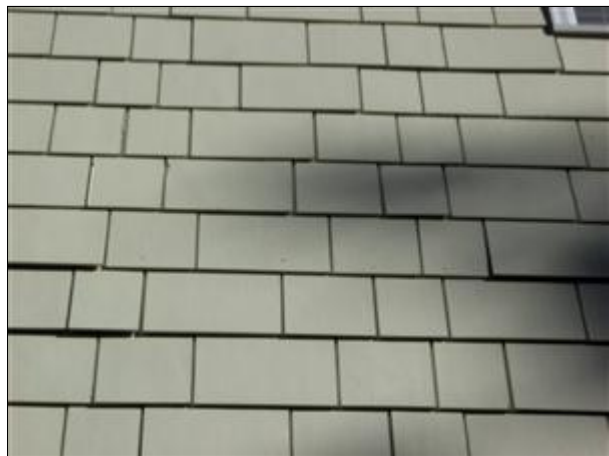
2.0 Picture 4 Left side above electrical panel
